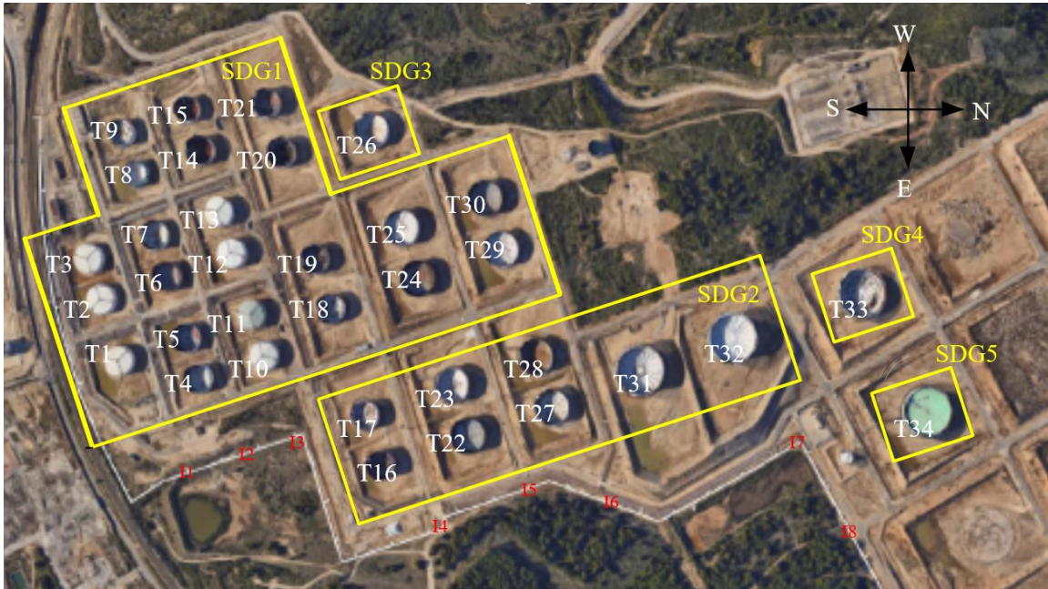
Fig. 6 Five domino islands within the chemical plant.
