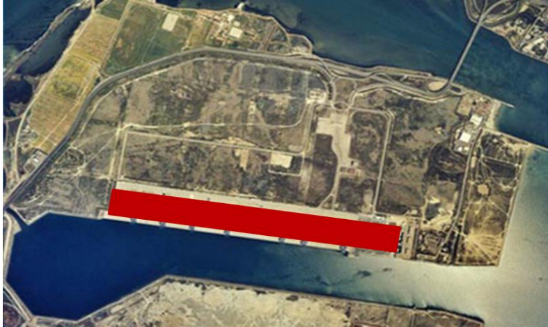
Figure 3. Structure of the Cagliari port
