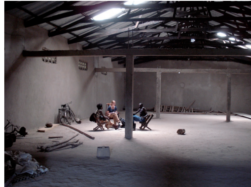
Newly constructed grain store, Acwec Omio Cooperative Society. Photo: Bill Vorley
