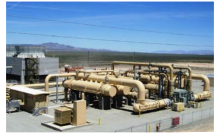
Binary Cycle elektriciteitscentrale, Beaver County (bron: http://www.cyrqenergy.com/projects/thermo/ )
