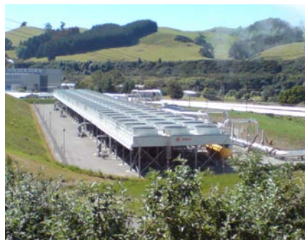
Geothermiecentrale Wairakei, Nieuw-Zeeland (bron: https://en.wikipedia.org/wiki/Wairakei_Power_Station )
