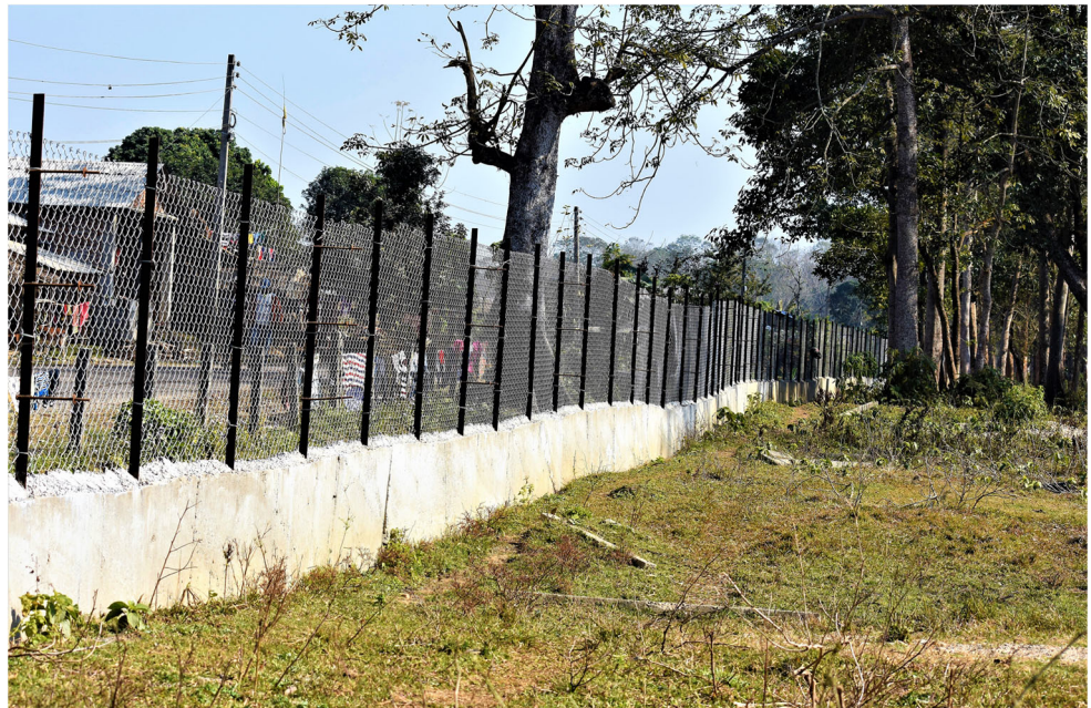
Fig. 7 An example of the mesh wire fence communities prefer to construct along the forest-settlement border. The fence has a concrete base of about 2 ft and 5 ft tall mesh wire anchored to the iron poles set in a concrete base
