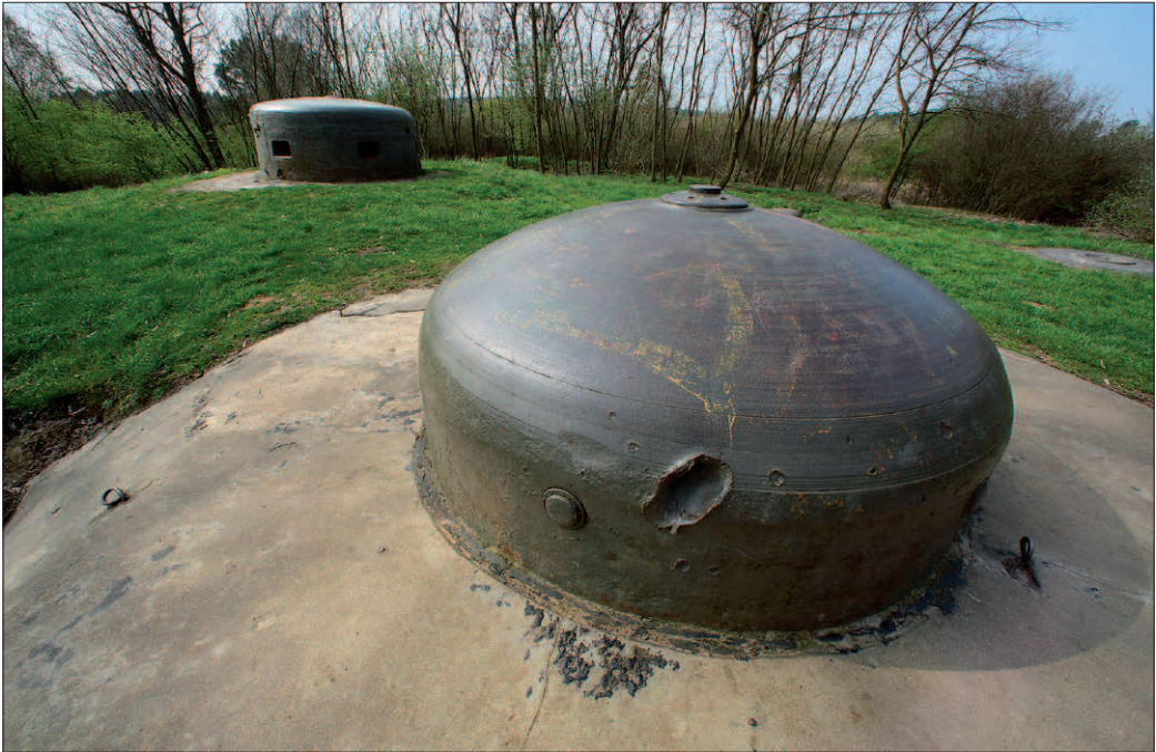
Fig. 1: Bunker PzW 716 – one of the entrances to the main underground system of „Nietoperek“ bat reserve.
