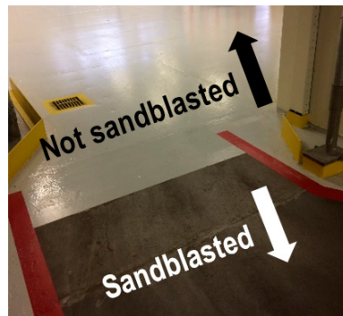
Figure 5. An example of a sandblasted and not sandblasted pallet mover transportation route.
