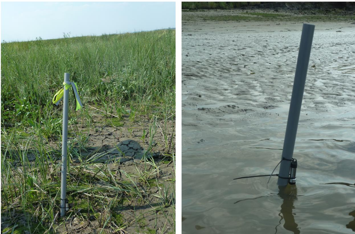
Figure 2.2: Water level loggers installed on the marsh platform (left) and in the marsh channel (right).
