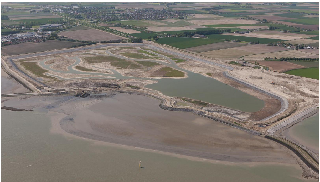
Creation of an intertidal area by de-embankment of the Perkpolder
