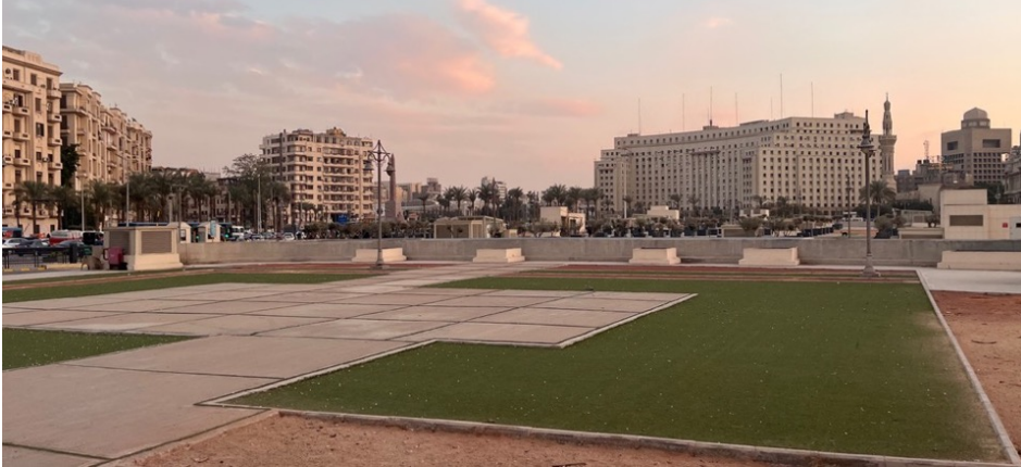
Figure 1: The roof surface of the subterranean garage in Tahrir with artificial grass. C: Mario Rinke. 2022
