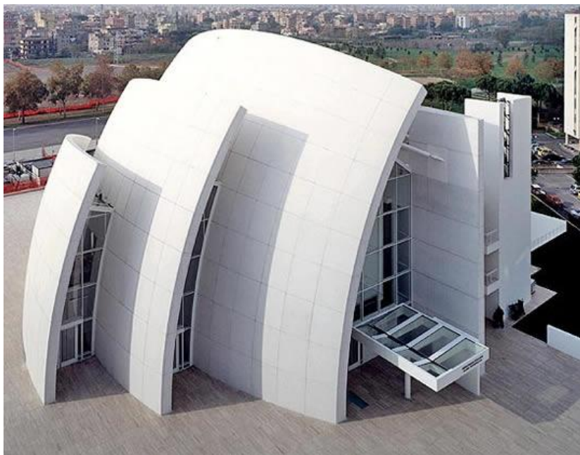
Figure 1.7. TiO 2 -based Jubilee church in Rome. Reprinted from Ref 96 with permission. © Elsevier (2010).
