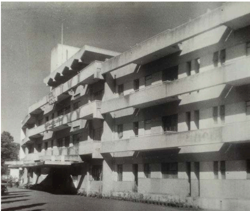
Figure 14: Interconnected parapets of aligned balconies were a common feature in modernist vernacular projects of the 1960s. Nehru Stadium Hotel, Pune, 1969, architect U. M. Apte. Source: private collection of Kiran Apte.
