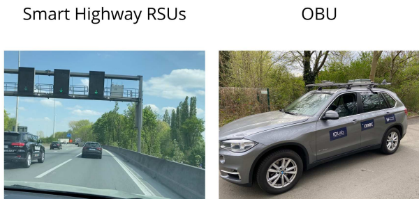
Fig. 4. Smart Highway RSU, next to BMW X5 equipped with ITS-G5 and LTE-V2X module
