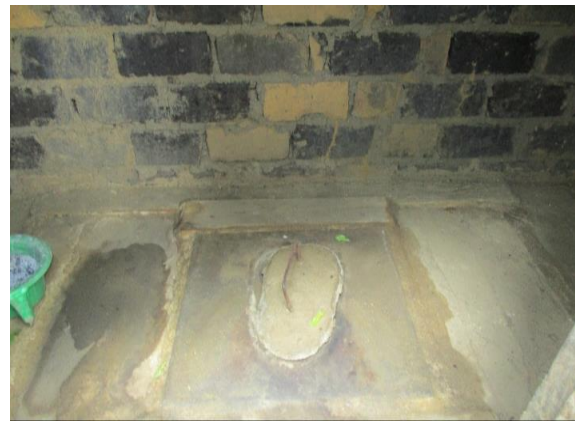
V5: A SanPlat slab toilet
