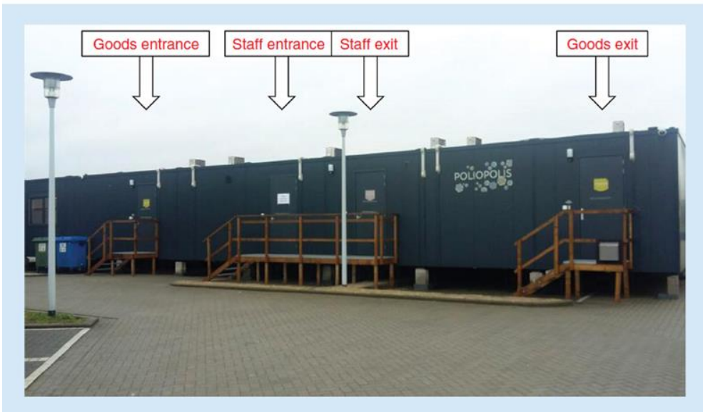
Figure 2. External appearance of Poliopolis showing the personnel entrance (left hand door) and exit (middle door) and the goods entrance and exit
