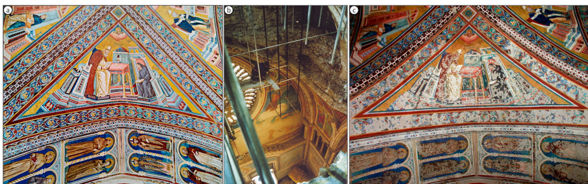
Figure 2. Photographs of the vaulted ceiling where Saint Jerome and the vaulting rib with the figures of eight saints were painted in the Upper Basilica of St. Francis in Assisi, Italy: (a) the outlook prior to the earthquakes in 1997, (b) view looking down through the ceiling of the nave after the earthquake (c) and after the restorations that ended in 2002.
