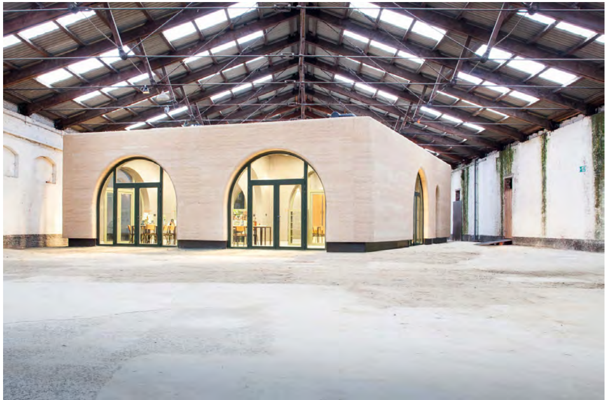
Figure 2: Fort V, Edegheem, Belgium, BC Architects & Studies, completed in 2018 (photography by Thomas Noceto).
