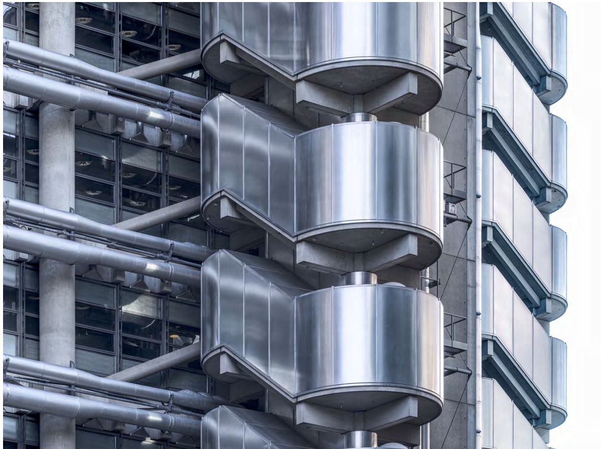
Figure 19: Detail of Lloyd's building, London, England, Richard Rogers & Partners, completed in 1986 (photography by Timothy Soar).
