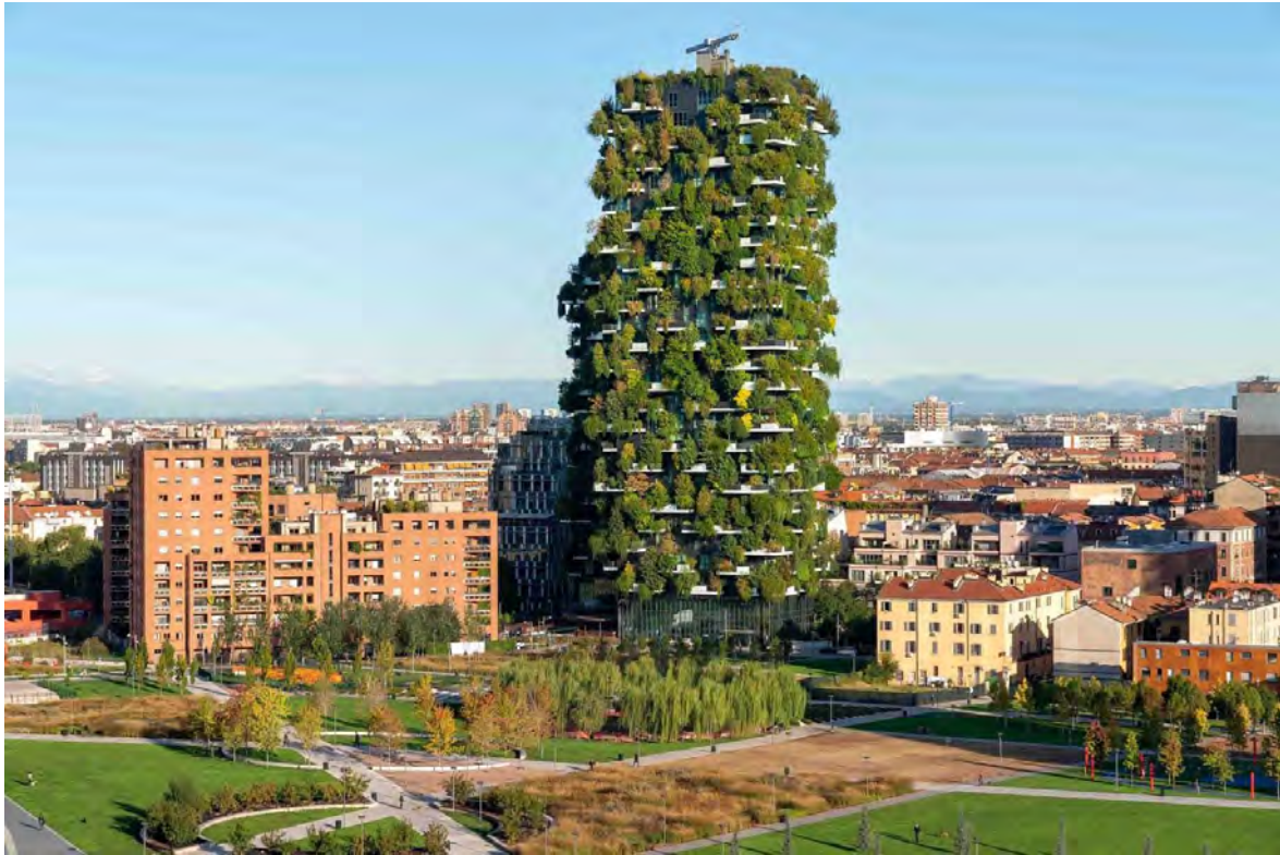
Figure 1: Bosco Verticale, Milan, Italy, Stefano Boeri Architetti, completed in 2014 (photography by Paolo Rosselli).
