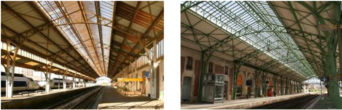
Figure 1: Gare de Perpignan, built in 1896, Perpignan, France (Pictures from SNCF-AREP by D. Boy de la Tour and A. Striffling). (a) Before and (b) after restoration of 2013.
