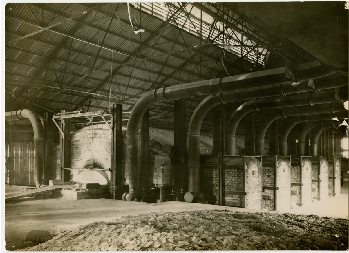
Figure 11: External view of a tank furnace
