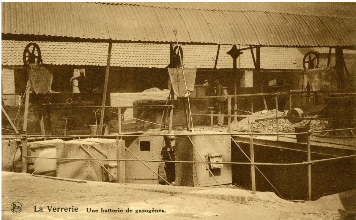
Figure 12: A battery of gas producers
