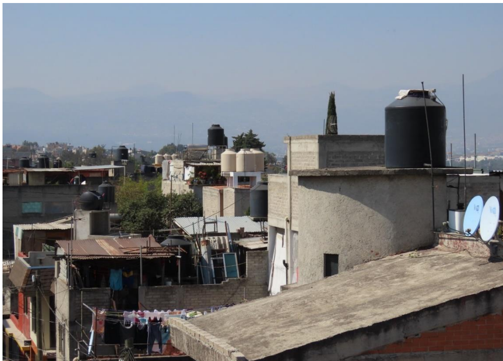
Figure 4: Water tanks (" tinacos " in Spanish) in Iztapalapa. Source: Author
