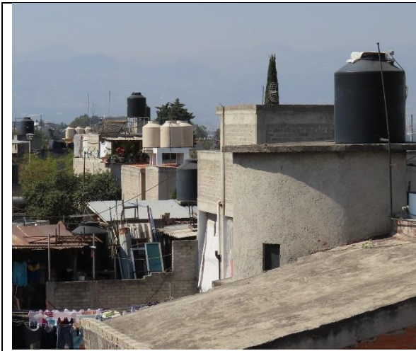
Figure 19. Water Tanks (“Tinacos” in Spanish) in Iztapalapa. Source: Author.
