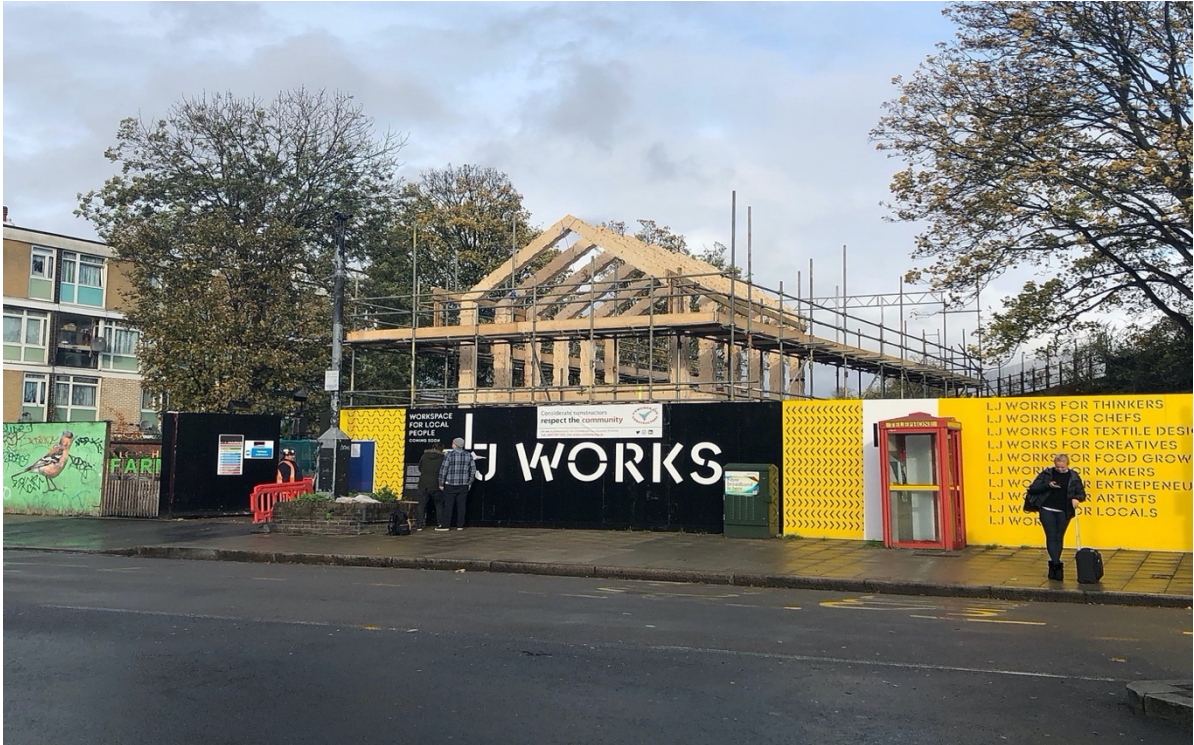
Figure 18. LJ Works under Construction
