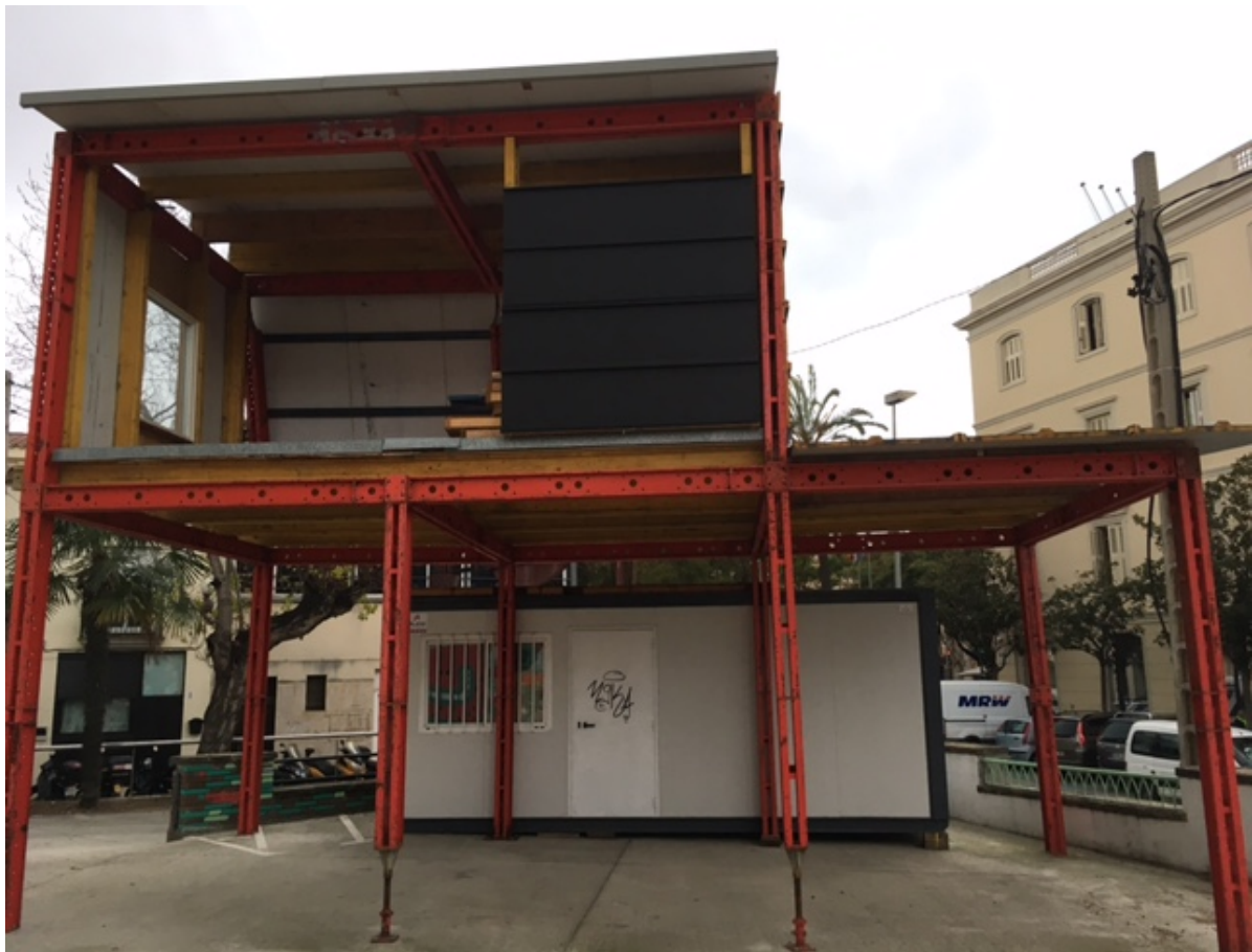
Figure 45. The Ateneu under Construction
