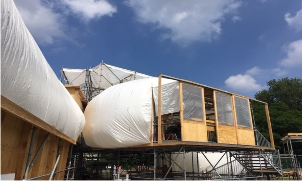
Figure 51. The Floating University under Construction
