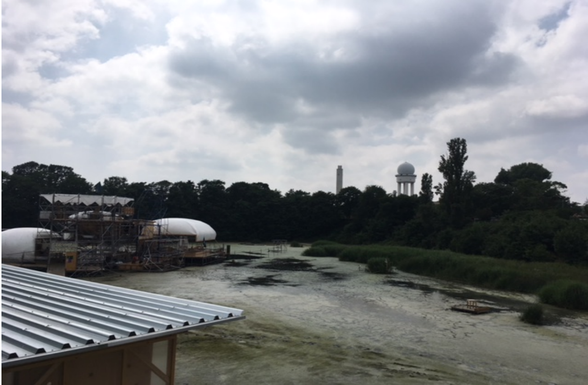
Figure 50. The Rainwater Retention Basin
