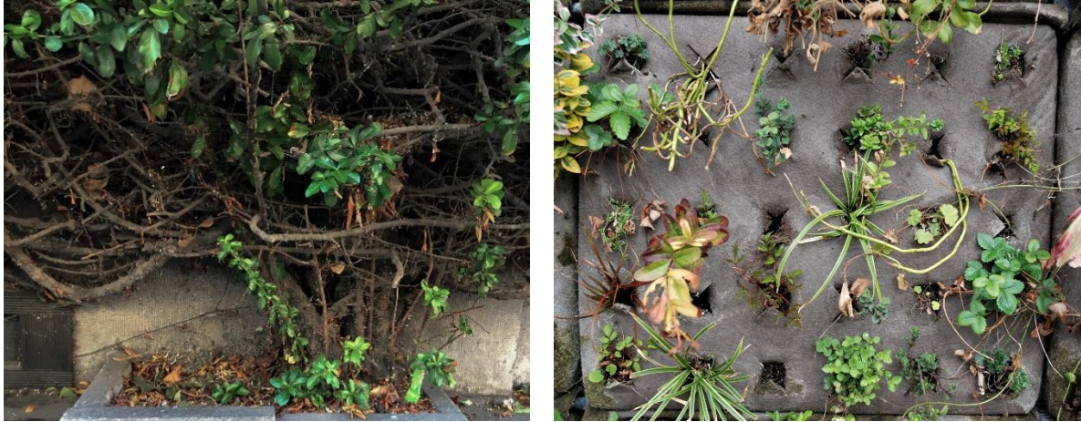
Figure 1: On the left a direct green façade (GF) and on the right a living wall system (LWS) placed in a city. Below these pictures, the rooting system of the GF and the support structure (here a panel made of rockwool) of the LWS.
