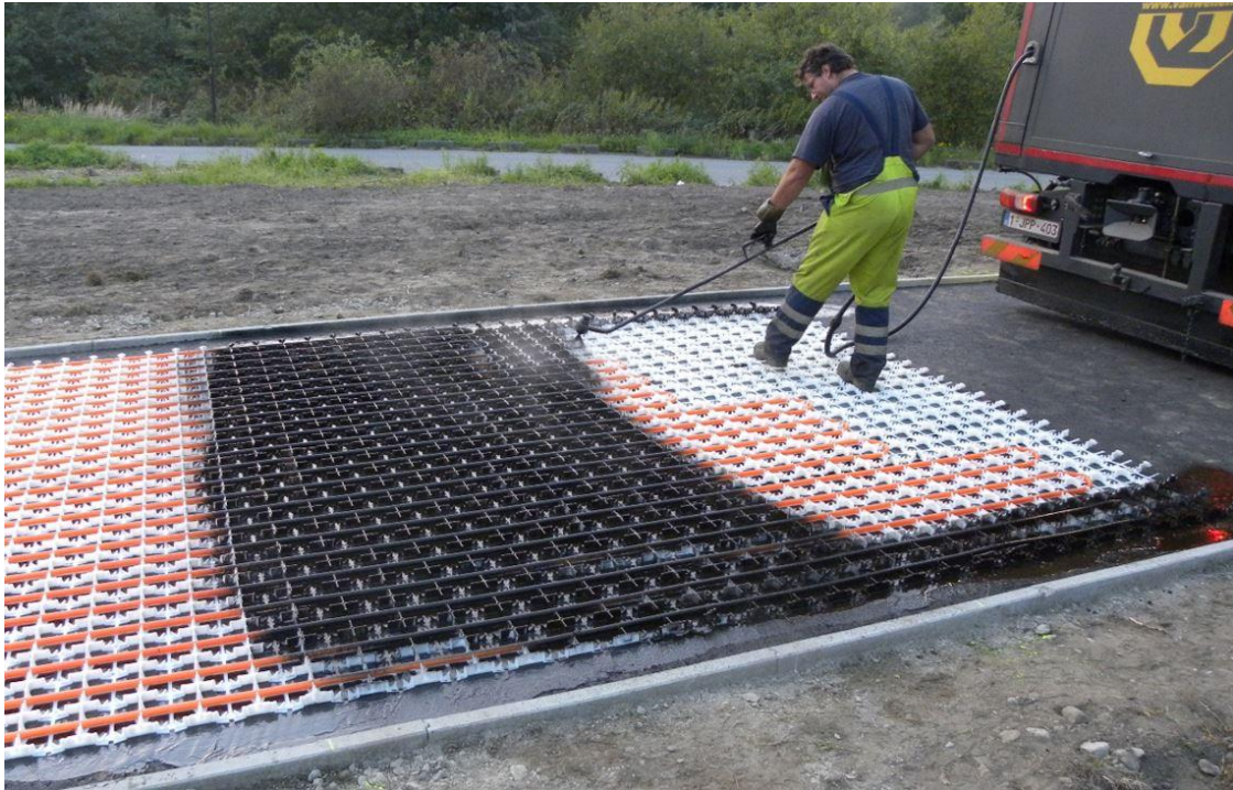
Figure 9. Spraying bitumen on the support grid and pipes before the asphalt placement [65]
