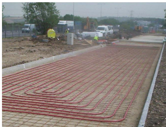
Figure 11. The construction stage of PSC without grid support (left) Power Road where the tubes are placed in grooves in the previously installed layer [67], (right) ICAX TRL project where the pipe network is connected to a steel square mesh using metal pins [45]
