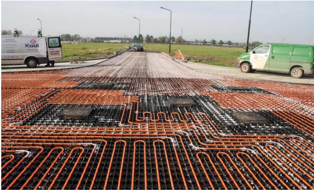
Figure 10. The construction stage of PSC with grid support in a RES project [115]
